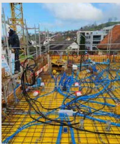
Neubau 2-FH in Herznach
